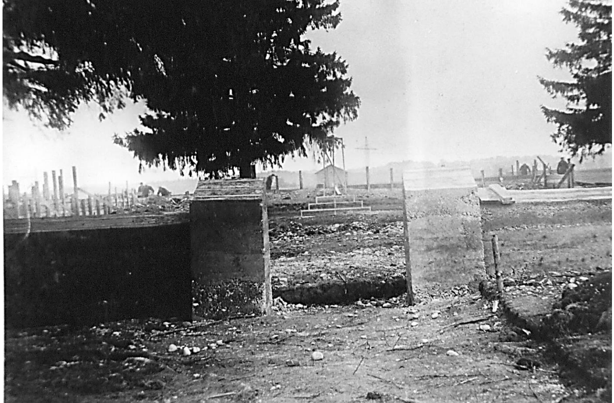
Image 8: Photo taken in May 1946, facing east. The western boundary wall with the entrance area is completed, while the remaining walls are partially formworked. The lattice framework for the central memorial stone has been erected. In the background, the power line to Kaufering is visible. Source: City Archives, Cemetery Files.
