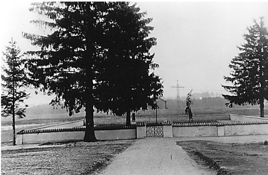
Image 8: Photo taken in May 1946, facing east. The western boundary wall with the entrance area is completed, while the remaining walls are partially formworked. The lattice framework for the central memorial stone has been erected. In the background, the power line to Kaufering is visible. Source: City Archives, Cemetery Files.
